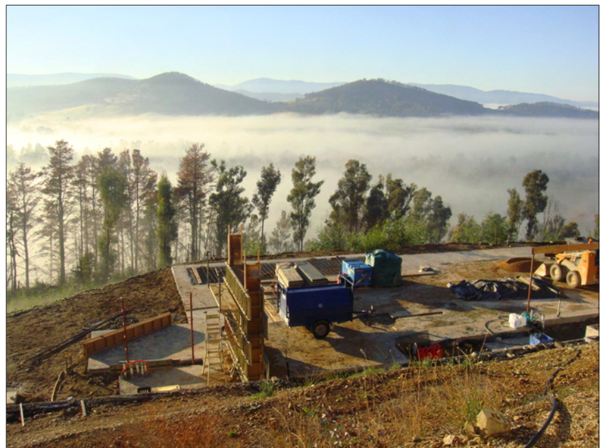
Early stages at the building site, where the old concrete slab was used for the rebuild.
