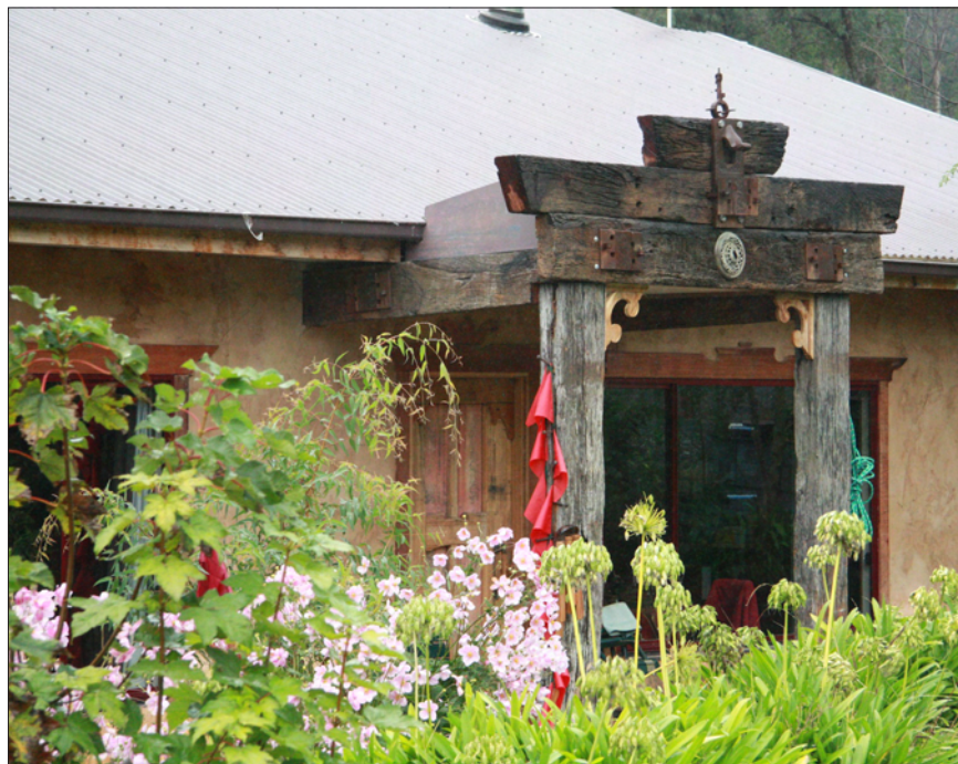
Cement sheet construction with an earth render help meet a BAL 19 rating.
